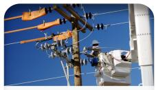
**SIF Workshop on Overhead Safety** Key focus areas include use of coverup, practices for gloving, practices for hotsticks, and technologies for worker protection. Hazards include contact, arc flash, step and touch voltages, induction, traffic, and falls.
