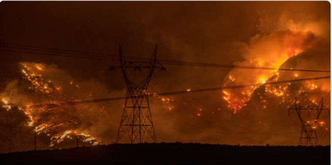
Distribution Asset Wildfire Performance Research on designing and maintaining distribution infrastructure, considering the risk of wildfire
