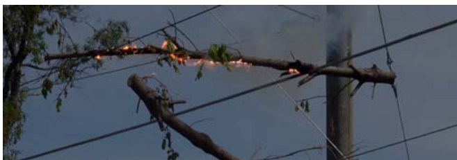
Figure 4. Limb across 12 kV conductors just prior to becoming a high-current fault
