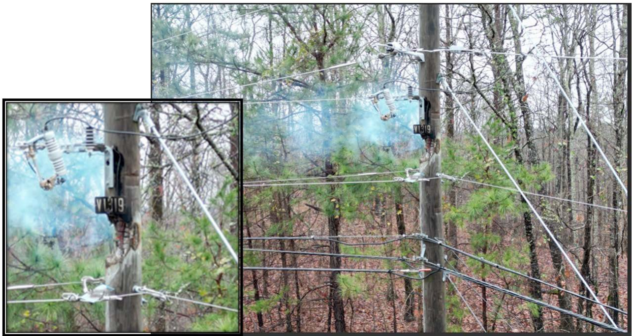
Figure 2. Active conductor to pole contact
