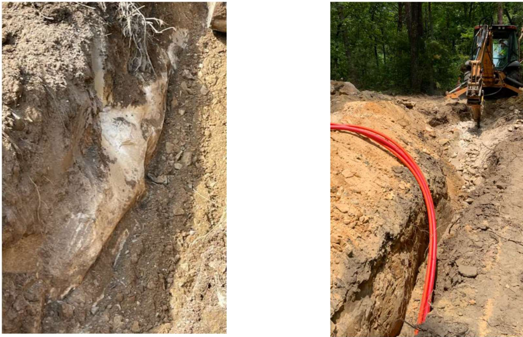
Figure A.13 Typical complicating geological factors for open trench installation
